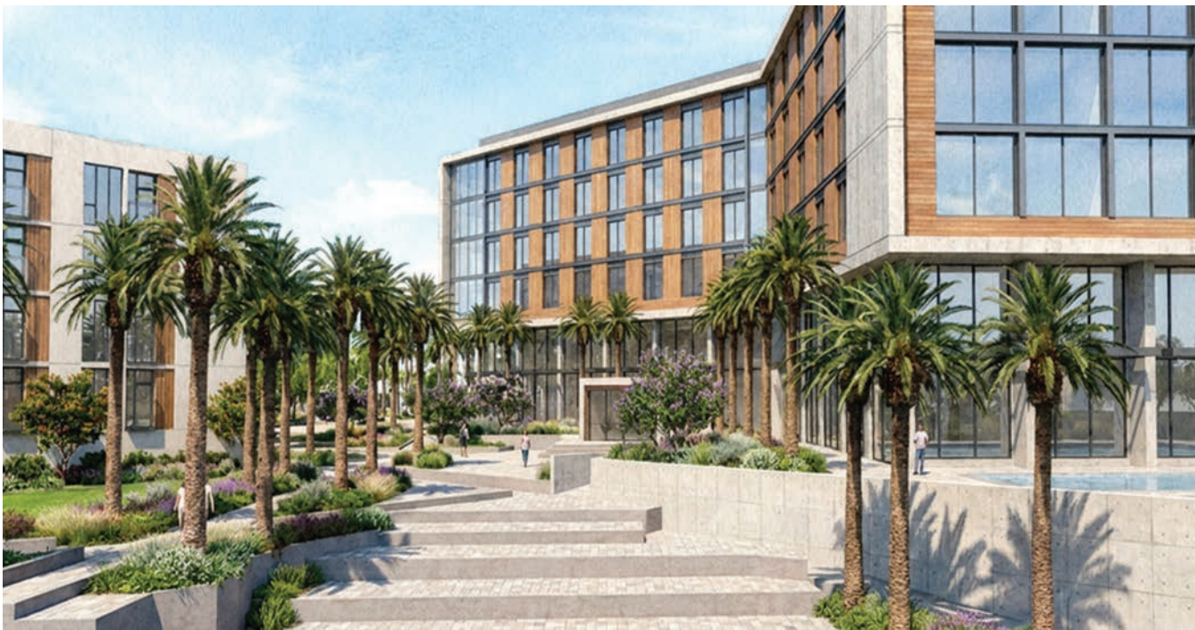
6. BASIN VIEW TO PARK AND HOTEL
