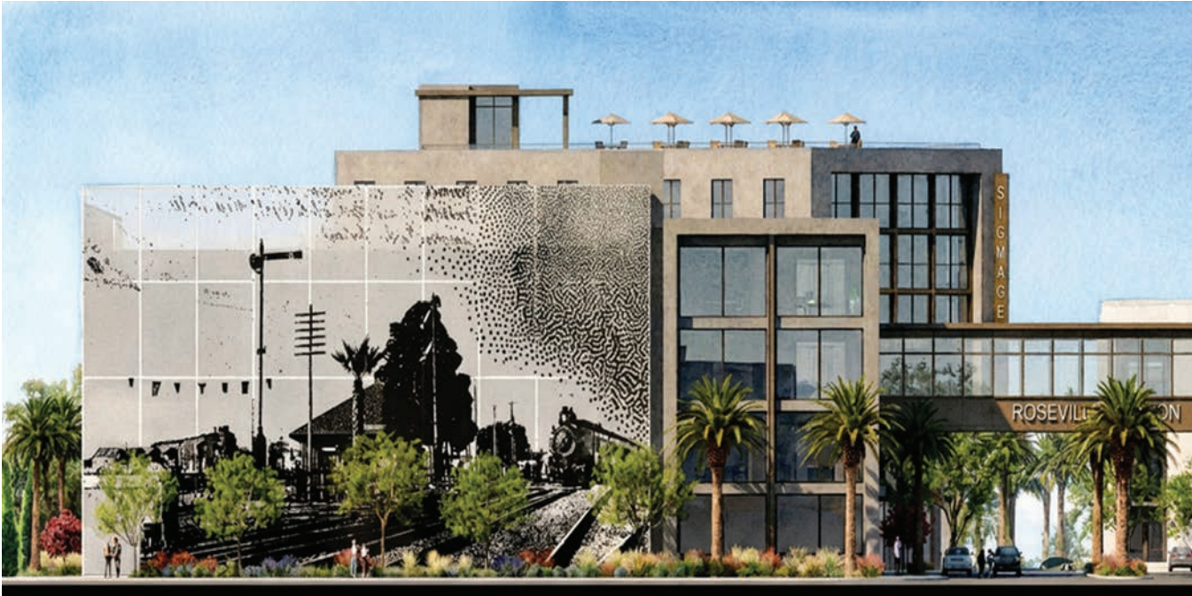
PARKING STRUCTURE + OFFICE BAR FROM GALLERIA
